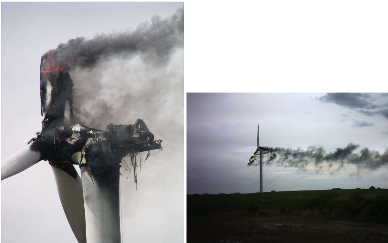
Fig. 1a+b: Fire after lightning struck a 2 MW wind turbine in 2004 (Image source: HDI/Gerling)
